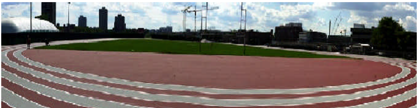
Surfacing of the outdoor track was completed in July, expanding it to 8 lanes of alternating red and gray.
